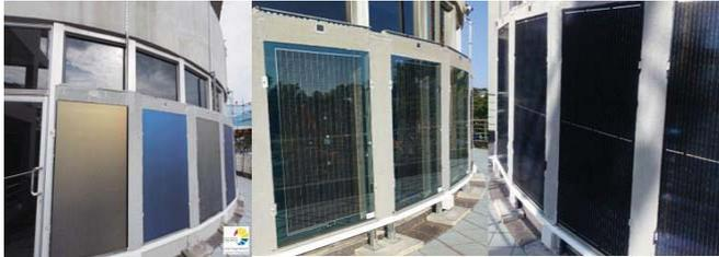
Figure 2. Architectural integration of various BIPV technologies.
