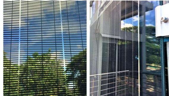
**Figure 3:** Original sample of semi-transparent BIPV: view from indoors (left), view from outdoors (right).
